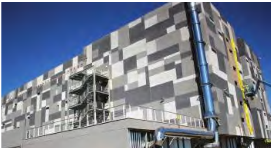
Chryso Southern Africa supplied an extensive range of products for the new Vodacom Business Date Centre in Midrand
