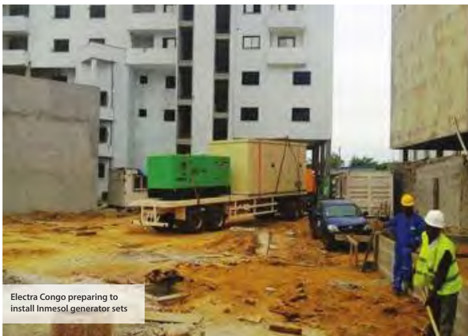
A series of parallel generator sets – IT720 and IT310 – can act either as the main supply or an emergency power source.
