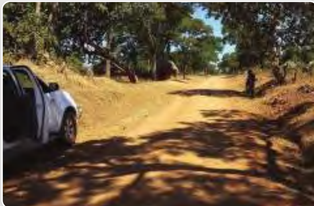
Louis Berger is assisting with the modernisation of the 350-kilometer-long, narrow and unpaved carriageway that crosses the Tete province in Mozambique
