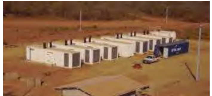
In Mali, SDMO has delivered a compliment of six T1900 sets in ISO40 containers
