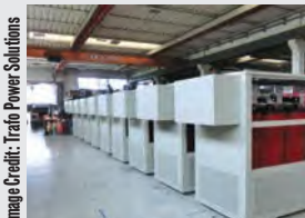
Trafo transformers will be used for a wastewater treatment plant near Vereeniging.
