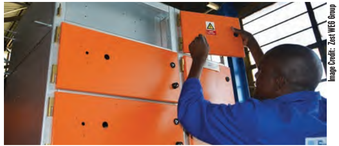
A live control voltage 110 VAC door being installed on a Shaw Controls aluzinc motor control centre.
