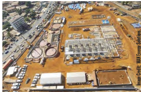
MAN Energy Solutions installs six MAN 18V32/40 engines with a total capacity of 53MW in a power plant in Conakry, Guinea.
