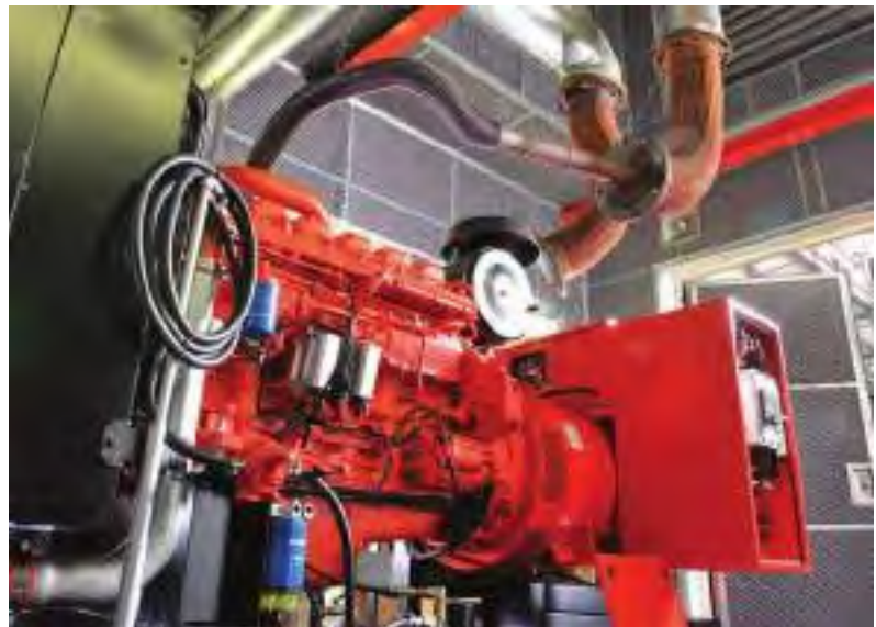
Open type diesel generator set
