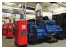
Six 2 000 kVA open type synchronising generator sets
