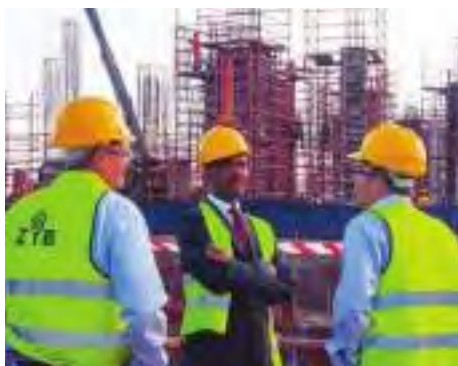
Zambia's Deputy Minister of Finance, Hon Christopher Mvunga, recently inspected construction of the US$32mn Zambian Breweries malting plant
