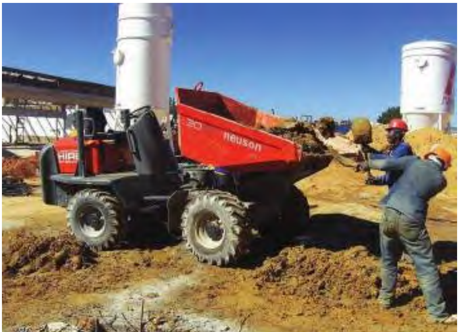
Hydrostatic drive unit concrete dumpers, available from Lambson's Hire, are ideally suited to the arduous operating conditions found on South African construction and building sites
