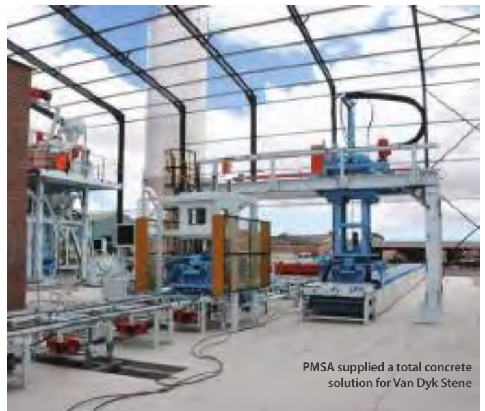
The Van Dyk Stene plant in Vredenburg, in South Africa's Western Cape
