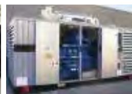
Containerised 1 250 kVA generator set
