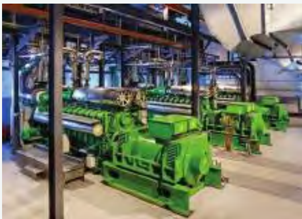
The Tronox Furnace Gas CHP Project at Saldanah Bay in South Africa
