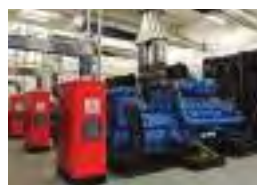
Six 2 000 kVA open type synchronising generator sets
