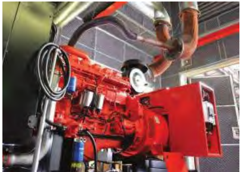
Open type diesel generator set
