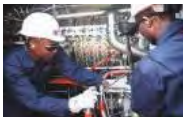
The new plant is expected to be commissioned in Q3 2015 (Photo: APR Energy)
