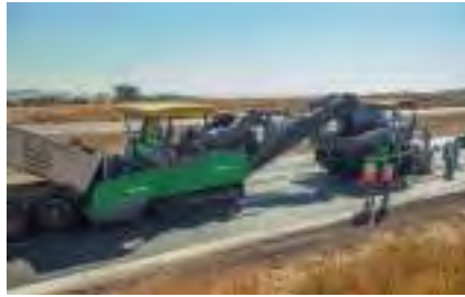
The VÖGELE material feeder works with the SUPER 1800-2 paver. (Source: VÖGELE)
