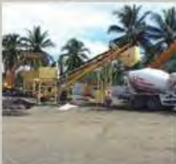
Dry mix concrete plant
