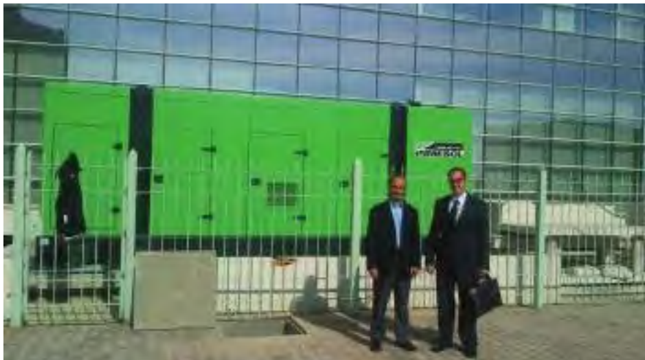
SEI manager Mourad Najjar and Inmesol sales manager for Africa José María Hernández in front of the equipment installed in Carthagène International Hospital Centre
