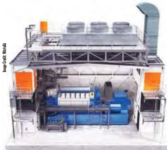
Four Wärtsilä modular block enclosures will provide 40MW to Resolute Mining's Syama off-grid gold mine in Mali.
