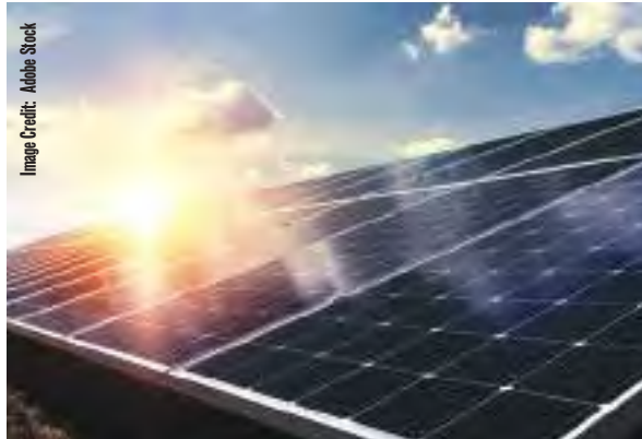
Scatec Solar will be supporting the Tunisian government's target to reach 30 per cent electricity via renewables by 2030.
