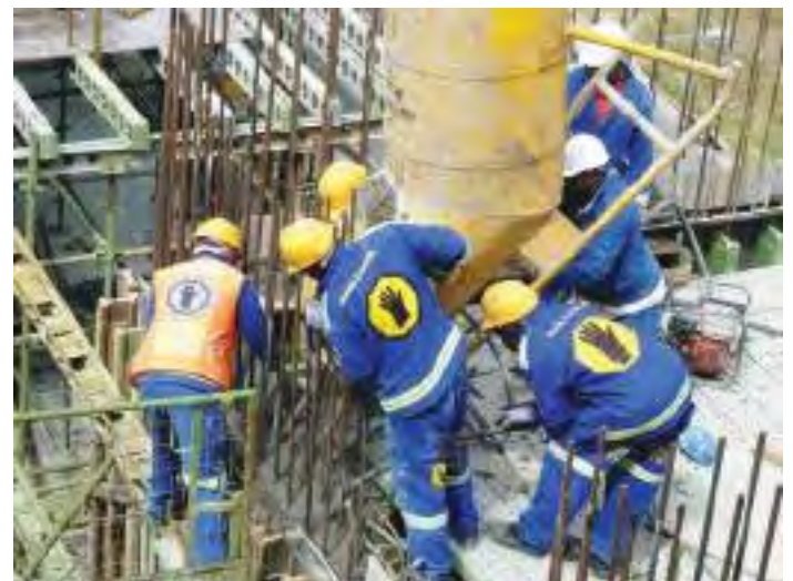
A concrete pour at Melomed Hospital. Murray & Roberts Western Cape used 6,000 m 3 of concrete on the project, which has a footprint of 3,000 m 2
