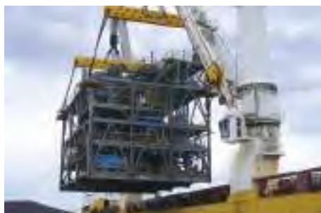
SNC-Lavalin focuses on engineering for simplicity of construction, which often means modularisation and containerisation
