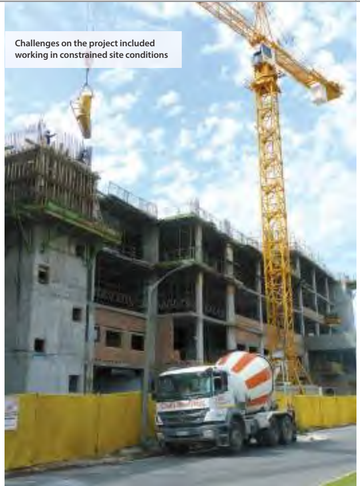
A concrete pour at Melomed Hospital. Murray & Roberts Western Cape used 6,000 m3 of concrete on the project, which has a footprint of 3,000 m2
