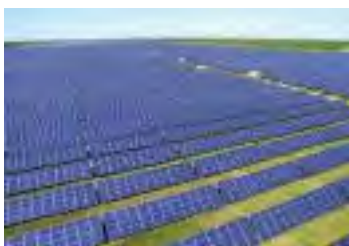
The university will spend US$750,000 to set up the laboratories (PHOTO: ActivSolar)
