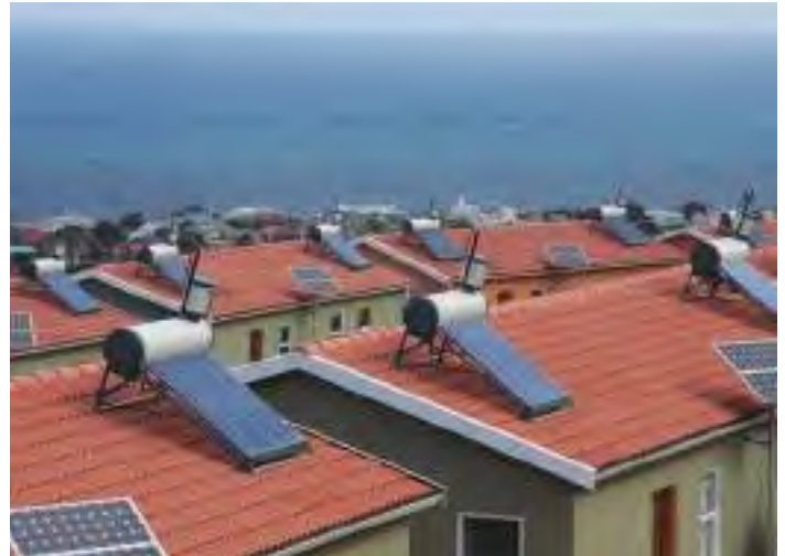
Technological breakthroughs have removed the hurdles from self-generation via renewables
