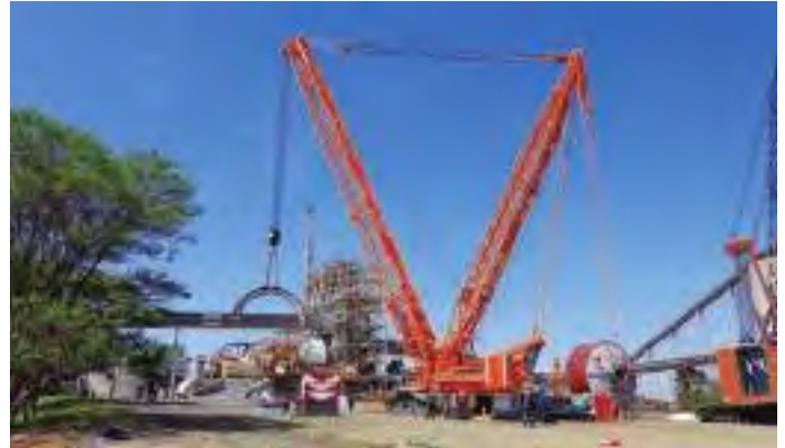
Johnson Crane Hire brought in a LR 1600/2,600t crawler crane from Europe to take off the gears, remove the old mills and install the new one at Zimplats' Selous Metallurgical Complex in Zimbabwe for client FLSmidth
