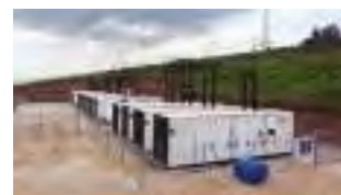
The SES 24MW rental power plant at Kigali, Rwanda. (PHOTO: Smart Energy Solutions)
