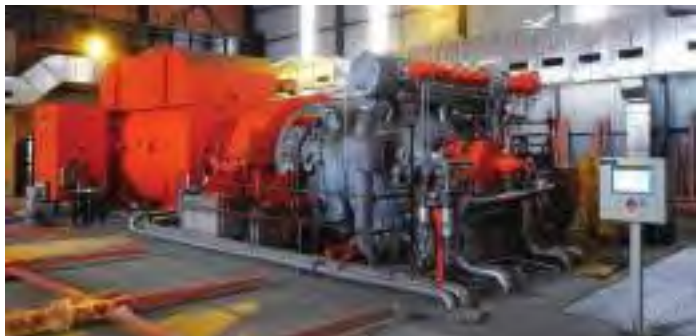
The steam turbo generator equipment during installation on-site. All major equipment had already been installed, with the thermal blankets just fitted around the turbine casing and the thermal acoustic hood in the process of being erected
