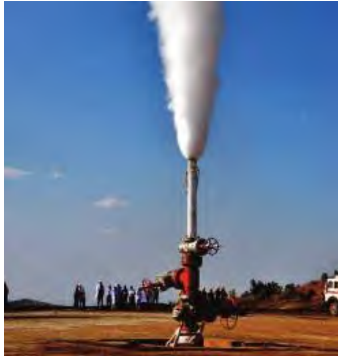
One of the discharging wells at the Menengai Geothermal Project (Source: Geothermal Development Company)
