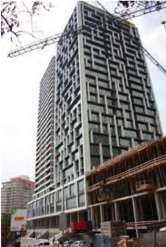
The Himoinisa Towers, Angola (Source: Himoinisa)
