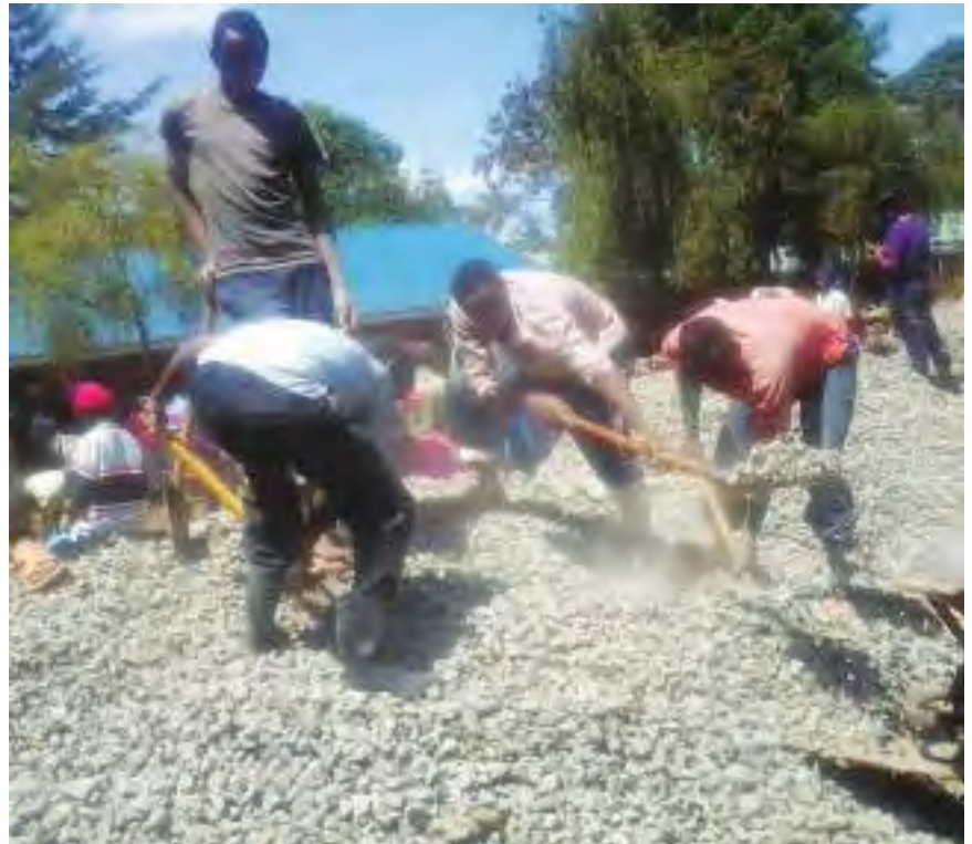
Masons and other workers on a construction site in Kenya (Source: Mwangi Mumero)
