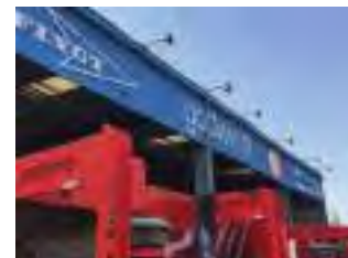
The expanded Tema Port harbour (Source: Aecom)
