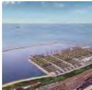
The expanded Tema Port harbour (Source: Aecom)
