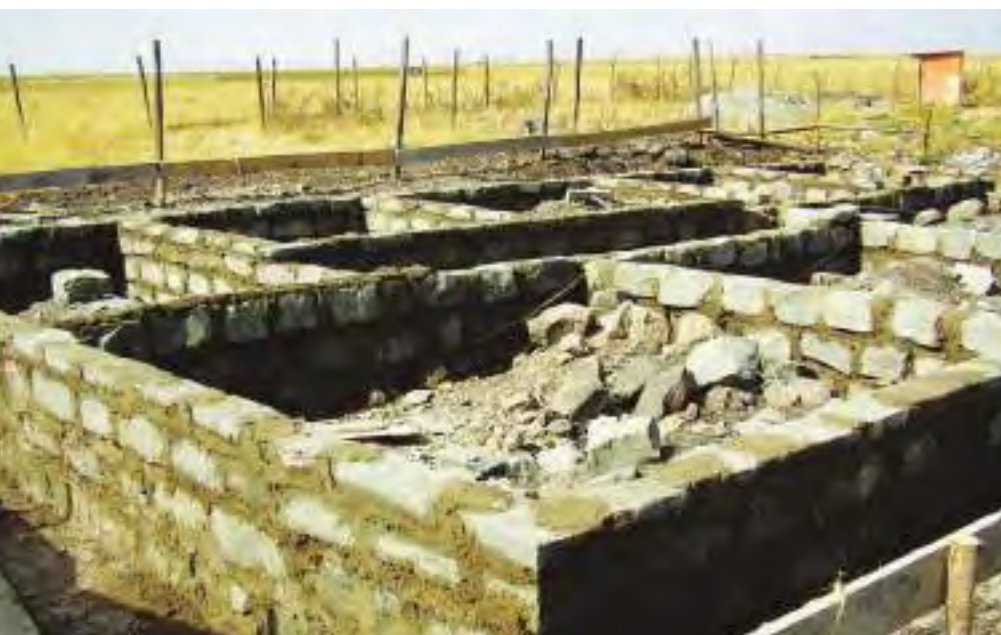
The foundations of an ongoing project (Source: Mwangi Mumero)
