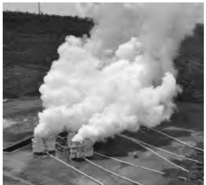
The 30MW well discharging at the Menengai Geothermal Development Project (Source: Geothermal Development Company)
