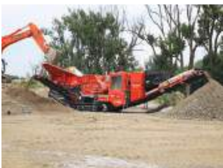
The Terex Finlay I-140 shows its performance in a recycling application
