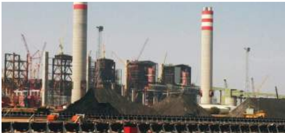
South Africa's mega 4,800MW Medupi Power Plant is still incomplete where costs have ballooned from an estimated US$4.34bn by Eskom CEO Jacob Maroga in 2007, to US$9.69bn today. (Photo: Wikimedia Commons)
