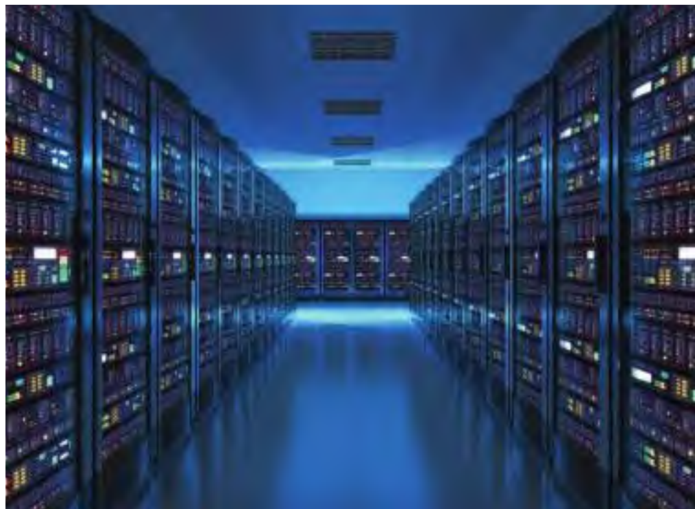
Kenya is currently the financial and manufacturing hub for the region and so possesses considerable demand from enterprise customers for data centre services (Image source: Oleksiy Mark/Fotolia)
