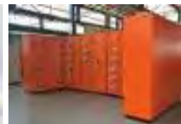
Motor Control Centres
