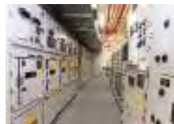
LV and MV Switchboards inside E-House
