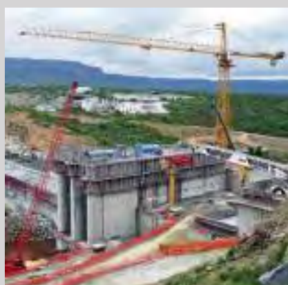
Potain tower cranes have moved material on many important civil engineering projects in South Africa
