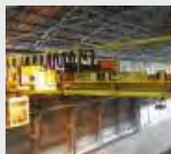
Demag's eight ton electric overhead travel crane
